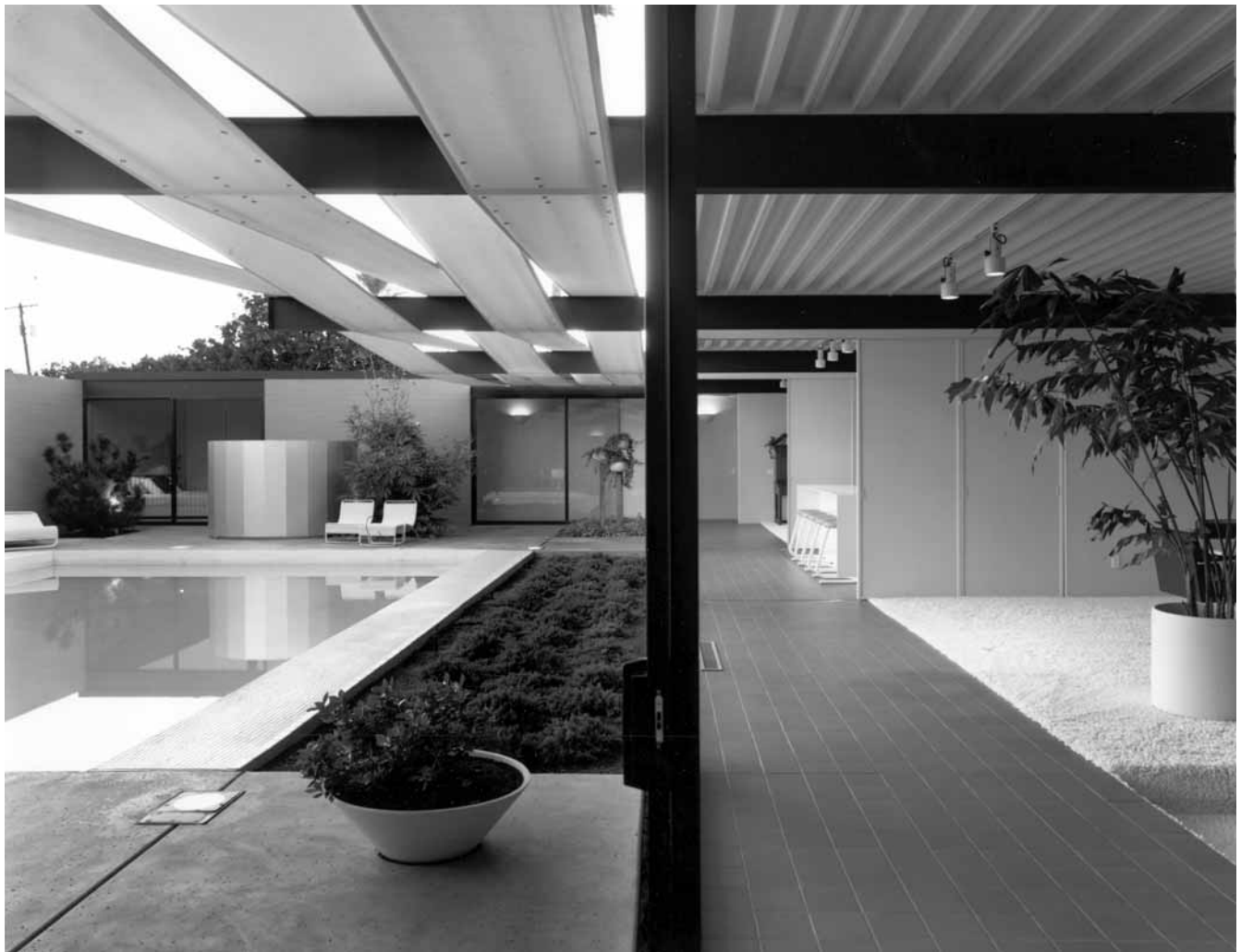
Above Patrick House, 1973, Scottsdale, Arizona. Beadle merged function and architectural grace in the sun shades, which were made of heavy mesh to allow for the passage of wind and rain.
