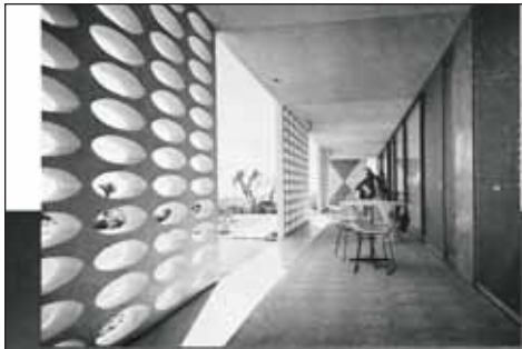
A malleable concrete screen filters sunlight and provides privacy for looking or looking on the larger which, actually, serves as a minimally-enclosed entrance, emphasized as a transitional zone by floor tags. It is also a structural point of circulation for the whole house. Sliding glass panels open to the living room, dining room, "small" room and bedrooms. Movable life guards are solar screens.
