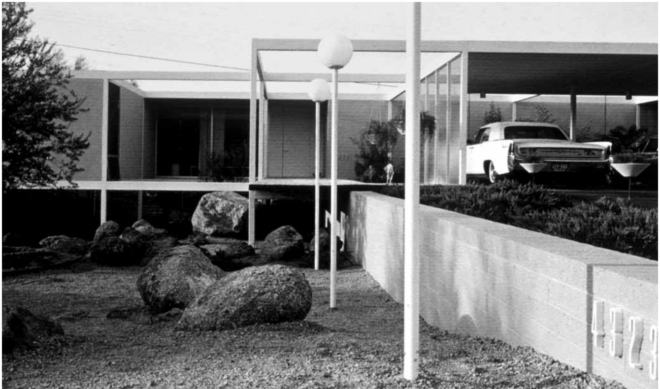
Above Beadle House 11, 1963, Phoenix. Beadle took full advantage of the desert landscape, building his family's home on a lot considered by most "a reject." The house, set on steel columns to raise it above the "wash" below, won a Design in Steel award from the American Iron and Steel Institute.
